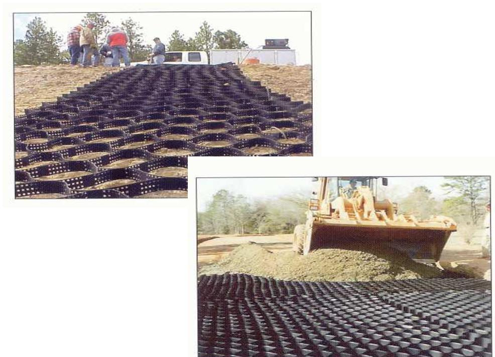
**Pictures show the Cell Web being installed on the ground.**
